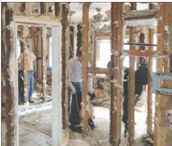
NYCDCC members at work ripping wet drywall and insulation from a flooded Staten Island home.
