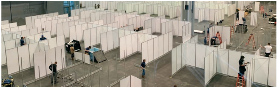
Our carpenters built over 1,000 hospital beds in under a week at the Jacob K. Javits Center to manage the overflow of patients at the height of the pandemic. In total, we built 2,500 beds.
