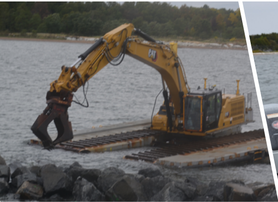
Swampcat excavator placing stones in specific formations
