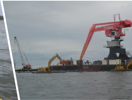
E-crane moves stones for the swampcat to access.
