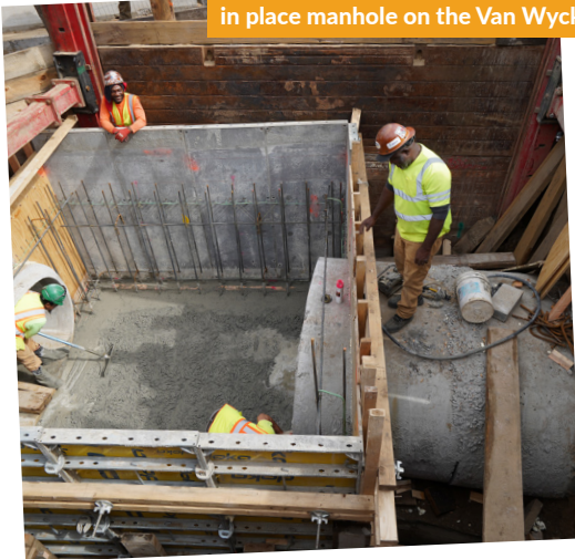
Local 1556 Timbermen work on a pour in place manhole on the Van Wyck
